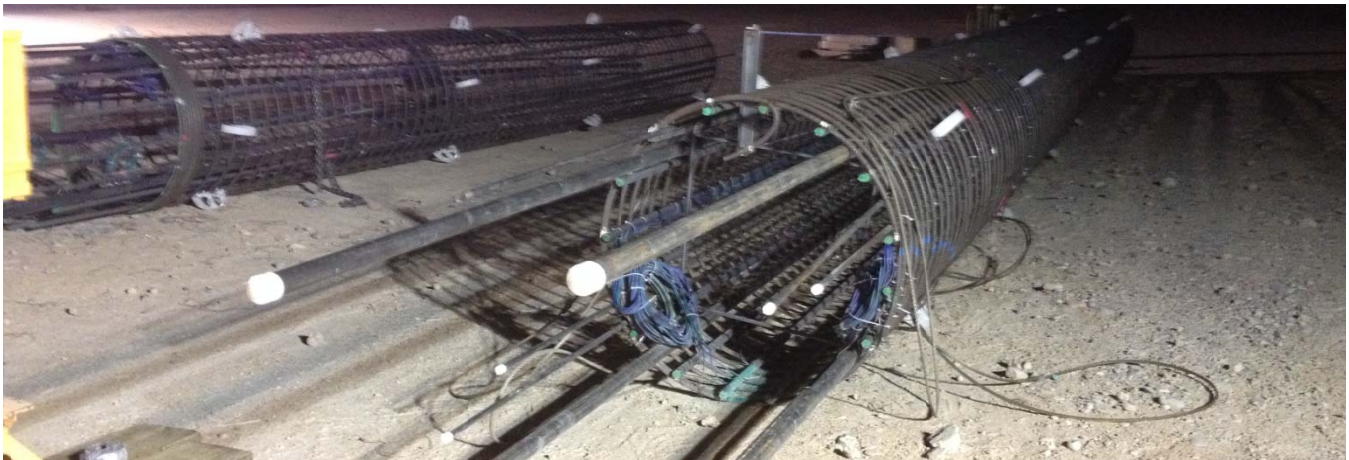
Shaft reinforcement with O-cell assembly.
